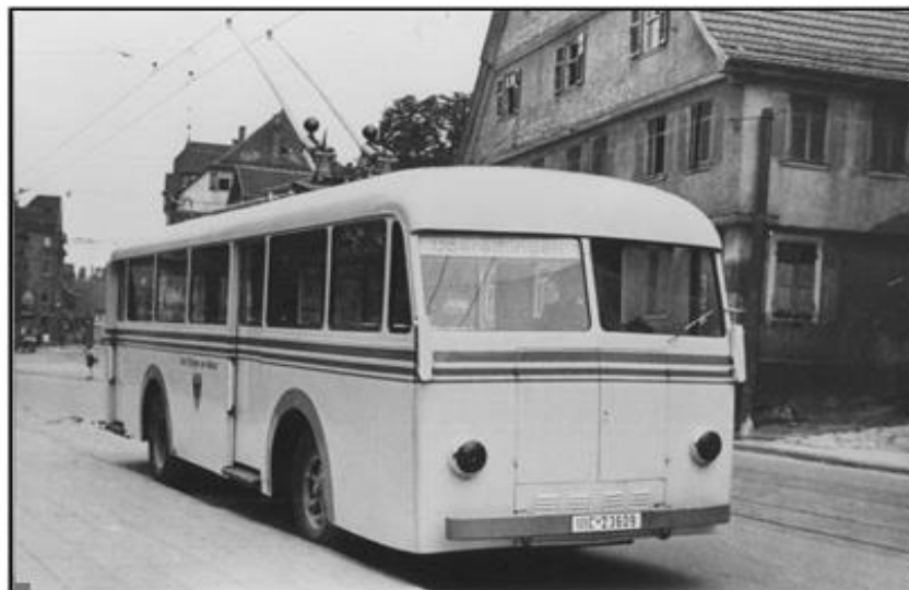
Figure 6. MAN MPE 4500 I/Kassbohrer/BBC trolleybus produced in 1944 with standard current collectors and camouflaged headlights in Esslingen (pictured late model on MAN MPE I chassis) (Kiebler, Ronald, 2000b).
