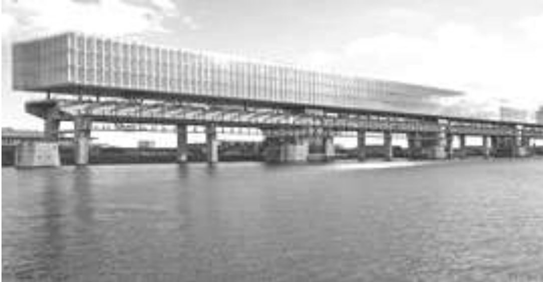
Figure 2. Kraanspoor office in Amsterdam
